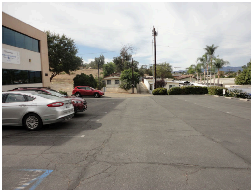
Asphalt paved parking lot
