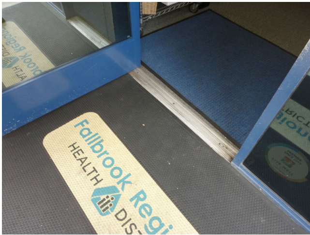
17. ADA compliant threshold
