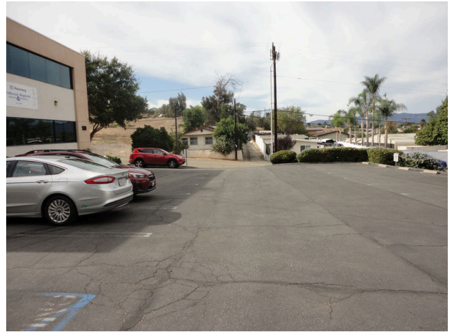
6. Asphalt paved parking lot
