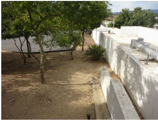
Retaining wall along north boundary
