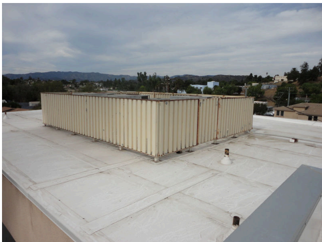
39. Overall view of roof
