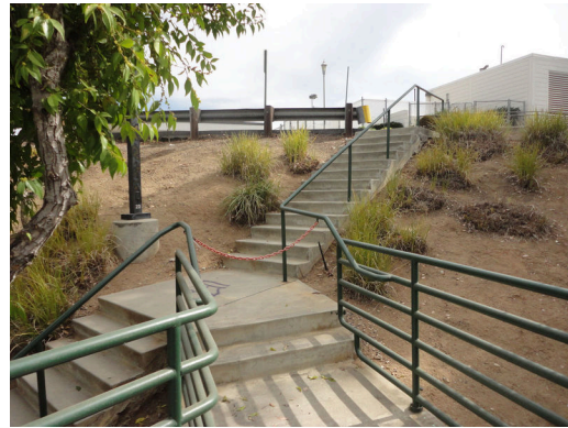
Concrete steps at east property line
