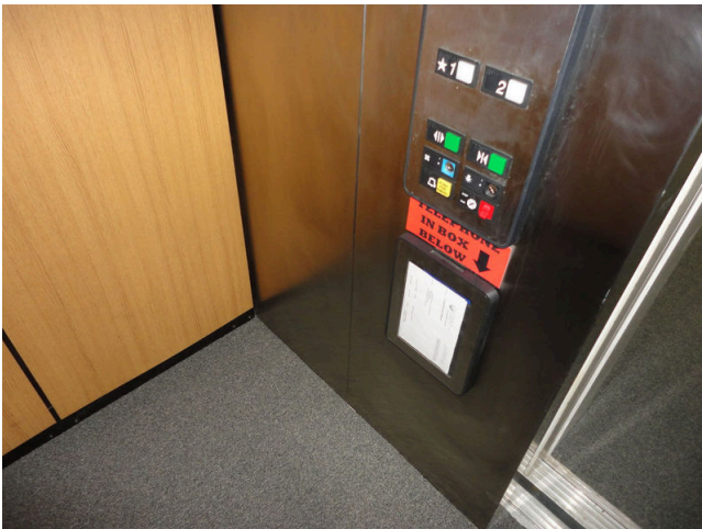
27. Interior of elevator
