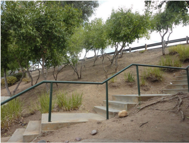
9. Concrete steps to east property line
