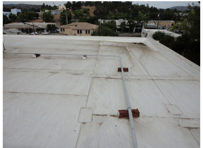
52. View of roof
