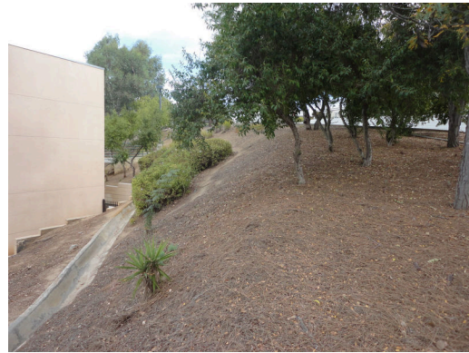
Drainage channel for slope
