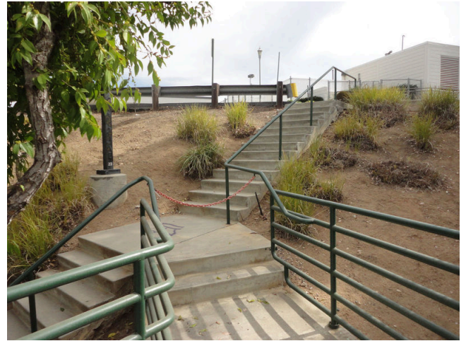
10. Concrete steps at east property line
