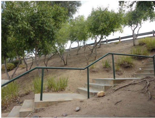
Concrete steps to east property line
