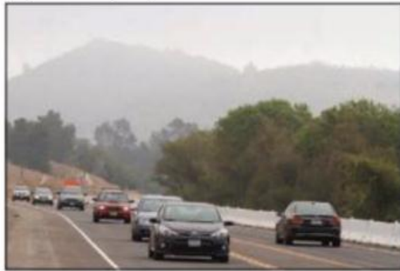
State Route 76 opens new eastbound lanes for traffic both ways.
