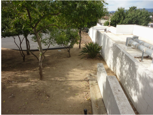
Retaining wall along north boundary
