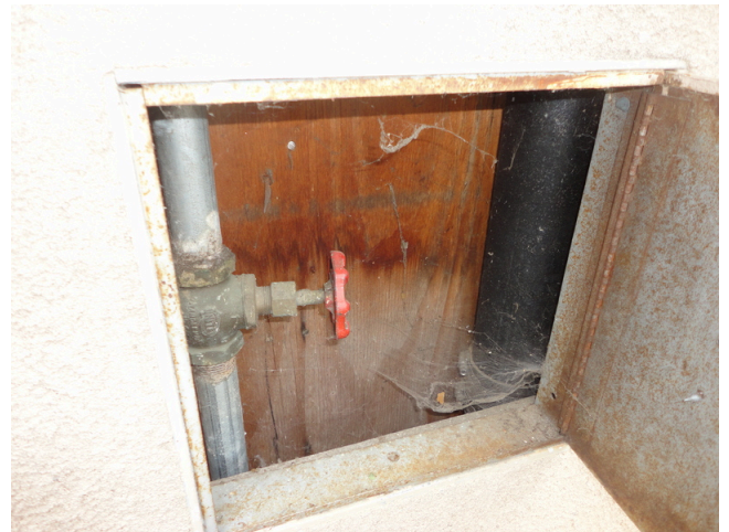
32. Water supply line
