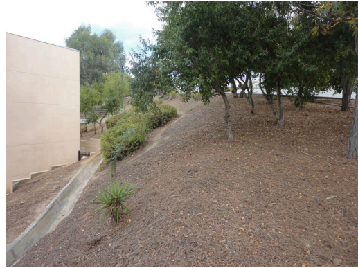
Drainage channel for slope
