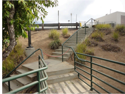
Concrete steps at east property line
