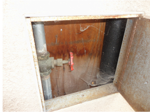
Water supply line
