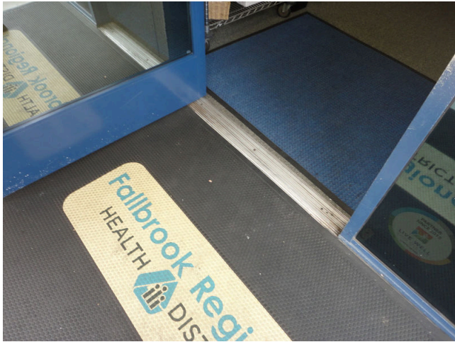
17. ADA compliant threshold
