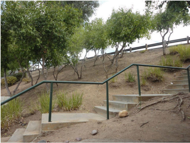
9. Concrete steps to east property line
