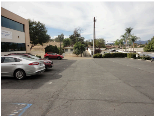
Asphalt paved parking lot
