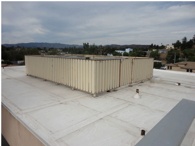
39. Overall view of roof
