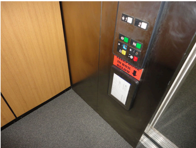
27. Interior of elevator
