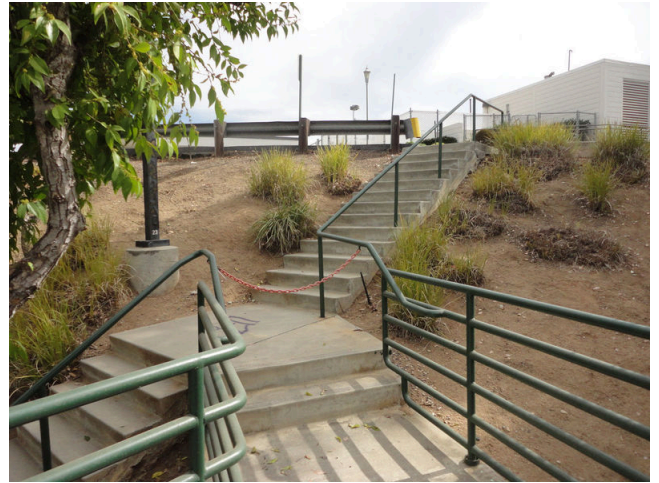
10. Concrete steps at east property line
