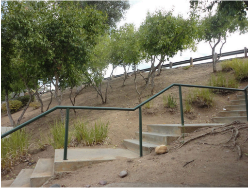
Concrete steps to east property line
