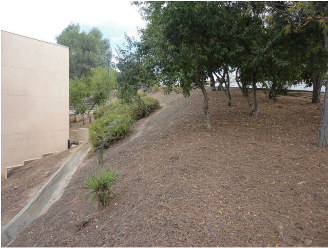
13. Drainage channel for slope
