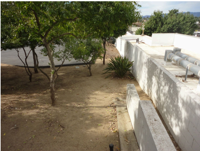
15. Retaining wall along north boundary
