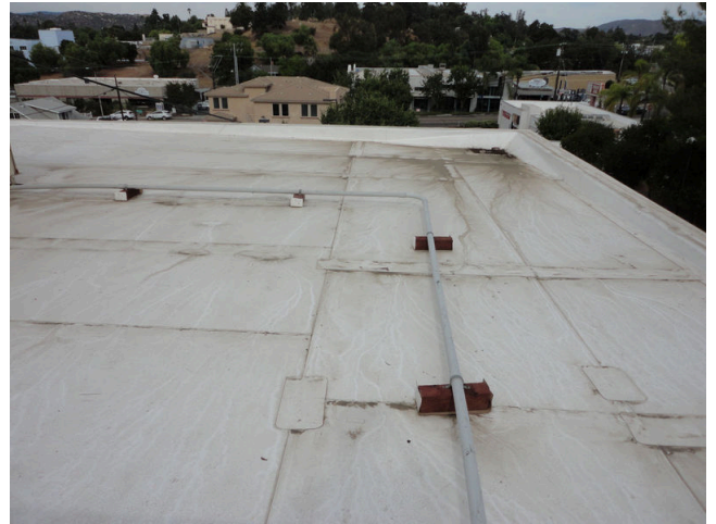
52. View of roof
